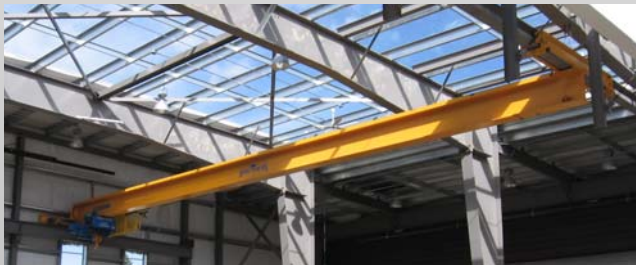
Top Running/Under Slung Overhead Crane. Far left is top running while the right side is under slung to achieve proper clearances.
