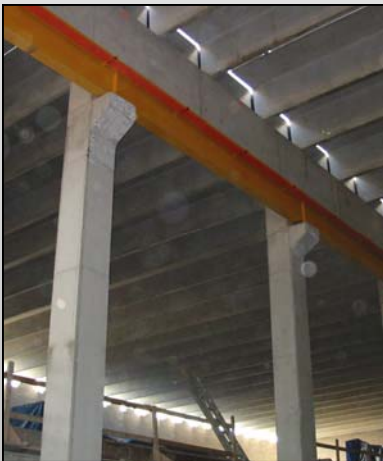
Installed Support Columns, Runways & Cranes at a water treatment facility.
