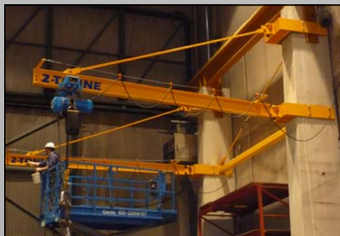
Tie-Rod style Jib Cranes mounted on concrete columns (below).
