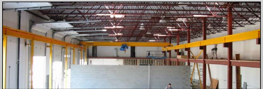
Tied-Back support columns for Crane Runway System (above).
